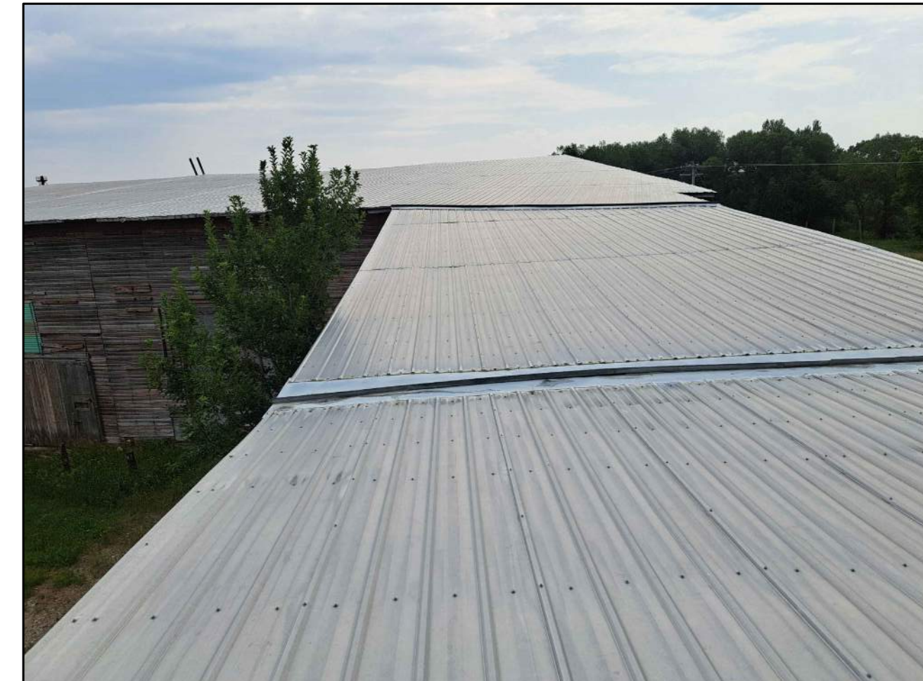
(E) ROOF LOOKING SOUTH
