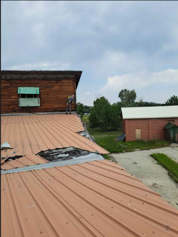
(E) ROOF LOOKING NORTH
