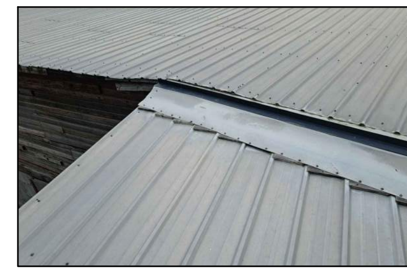
(E) NORTH ROOF VALLEY CONDITION, SEE DETAIL 7
