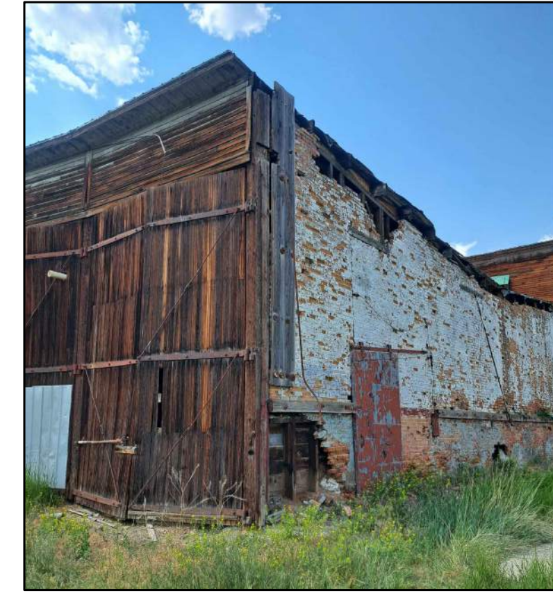
(E) NORTHEAST ROOF CORNER & (E) EAST WALL
