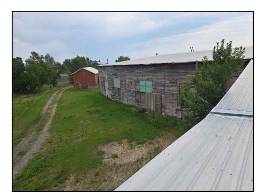
NORTH WALL AND ROOF
