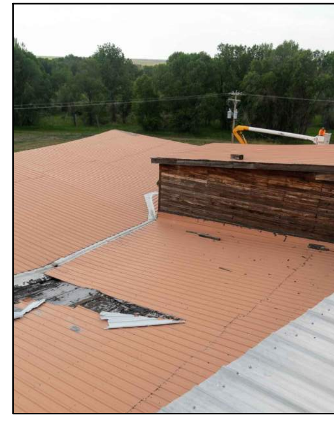
(E) ROOF DRAIN CONDITION, SEE DETAIL 6
